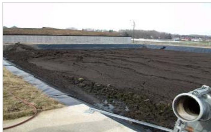
Figure 15. Storage of digested residue after anaerobic fermentation (Biogas plant in Austria)
