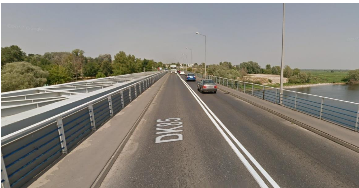
Picture 5: The Feliks Pancer bridge over the Narew river
