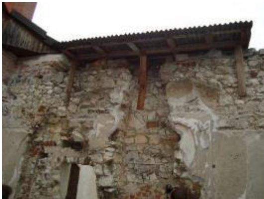
Photo 93 South arcades: roofing above moulding
