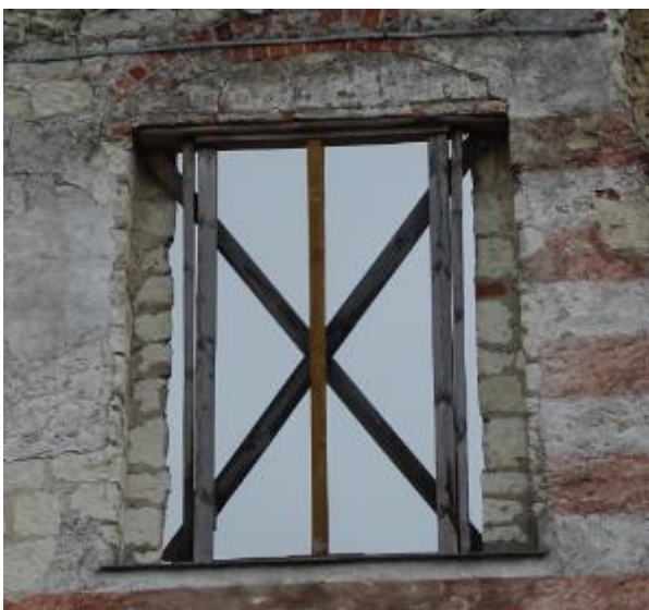
Photo 42 Temporary strengthening of lintel with wooden elements
