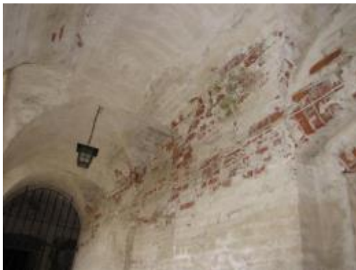
Photo 100 East wing: interior plaster
