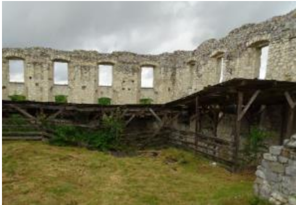
Photo 76 Wall coping protection in excavated basement: wooden roofing
