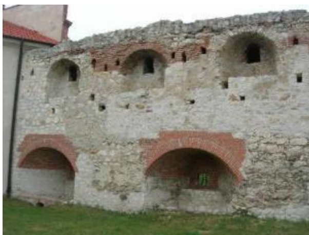
Photo 36 North wall - strengthening improvements with non-original masonry material
