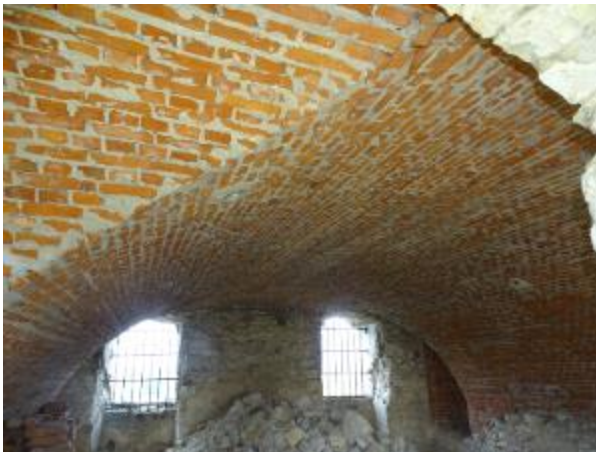
Photo 40 Non-original ceramic brick - strengthening improvement of vaults and ceilings
