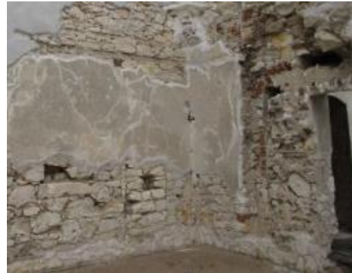
Photo 103 South suite of rooms: plaster protection
