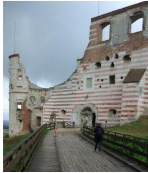
Photo 52 Gate house facing the bridge; 2017.
