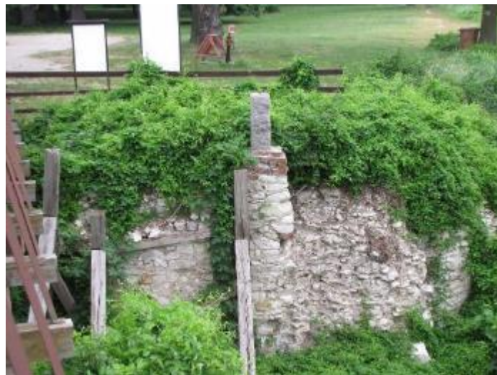
Photo 113 The moat facing the bridge
