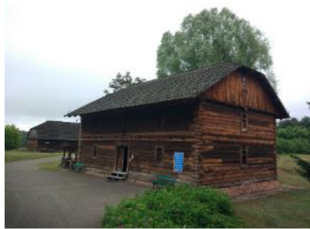
Photo 33 Granary of Podlodów
