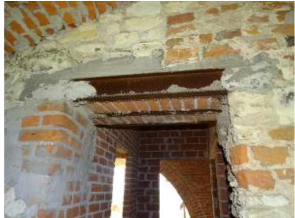
Photo 39 Installing steel beams in the existing wall
