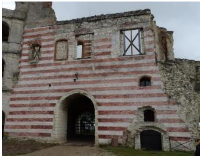
Photo 50 Gate house facing the courtyard; 2017.
