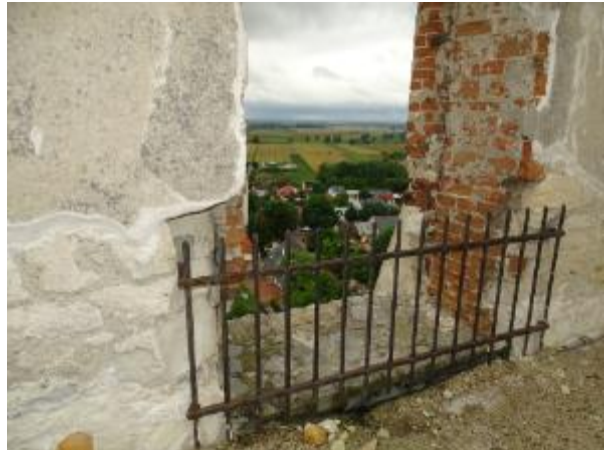
Photo 22 Access restriction rails
