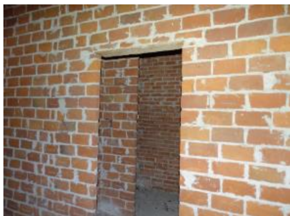
Photo 61 Dividing walls made of ceramic solid brick - non-original material
