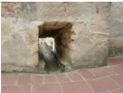
Photo 84 A gargoyle conveying water from profiled floors
