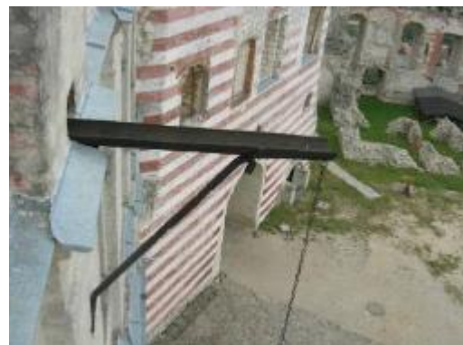
Photo 85 Gargoyles conveying water away from the building onto the courtyard
