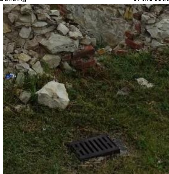
Photo 90 Drain grate located above grade
