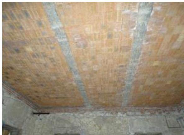
Photo 60 Replacing ceilings with contemporary Ackerman ceiling installations.
