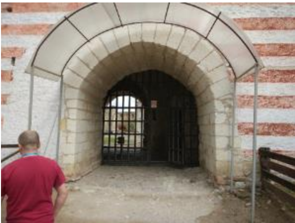
Photo 23 Protection roofs above the entrance to the castle
