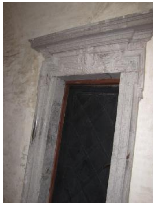
Photo 92 Baroque-style marble portal; first floor in east wing
