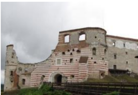
Photo 98 Gate house: re-plastering of a part of the face of walls; reconstructing decorations according to elements that remained from the past
