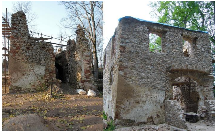
Figure 14 Restoration of captain's residence at Castle Muráň
