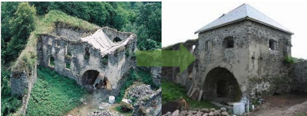
Figure 7 Gate no. II of Castle Čabrad' - restoration done by local civic association Rondel.
