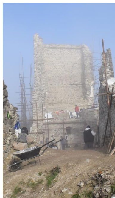
Figure 18 Restoration of the main tower of Castle Revište
