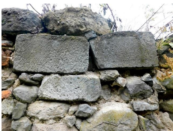
Figure 24 Chiselled blocks in the wall structure
