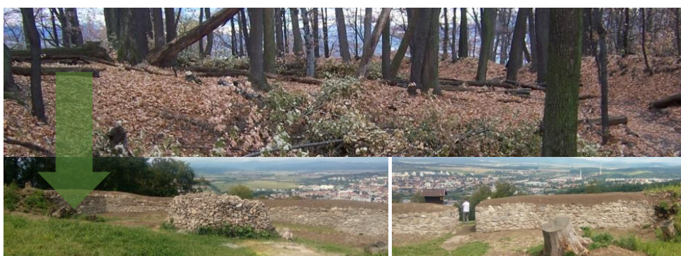
Figure 13 Restoration of the ramparts of Castle Pustý Hrad
