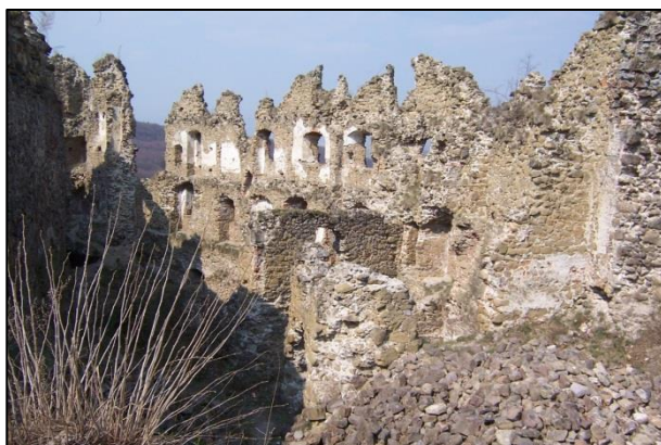
Figure 6 Ruins of Castle Šášov – situation after stopped restoration process, where the ruins were cleaned of the rubble and total archeological excavation was finished. Then the ruin was left to the elements.
