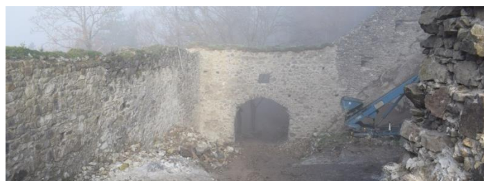
Figure 16 Restoration of the gate no. 1 and clean-up of rubble coming from a massive wall collapse into outer courtyard at Castle Revište
