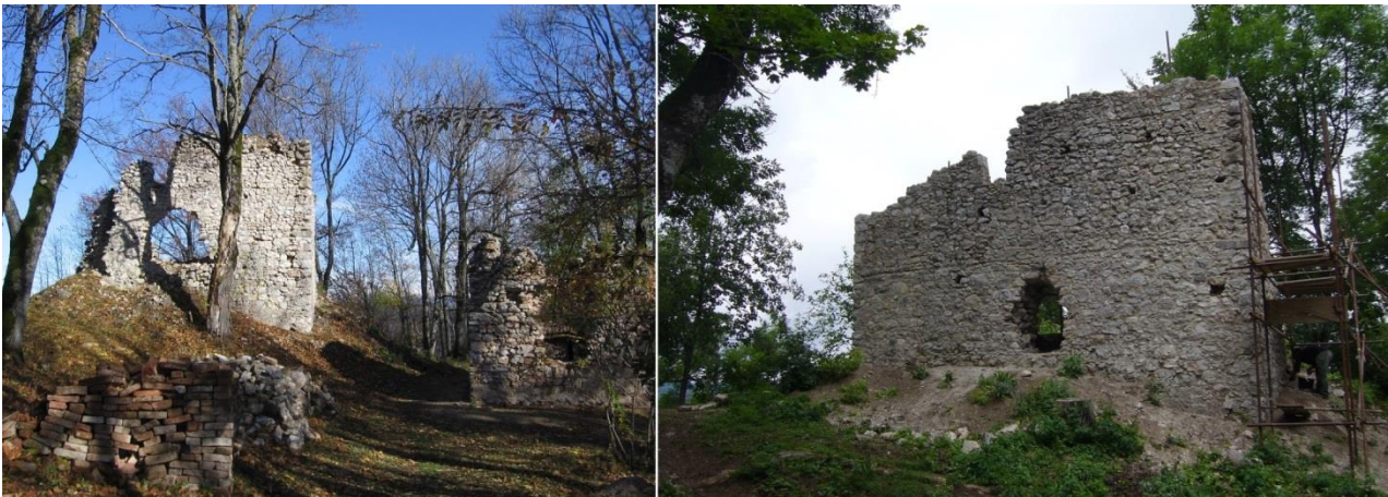
Figure 15 Restoration of the main tower of Castle Muráň
