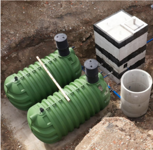
Pilot plant building. Photo: Aleš Erker, MBVOD.
