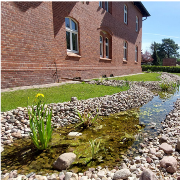
Rain gardens at Waterworks Museum in Bydgoszcz. Photo: Jacek Cieściński, Bydgoszcz Municipal Waterworks.
