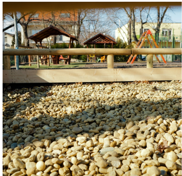
Filter gravel bed. Photo: Zugló Municipality.
