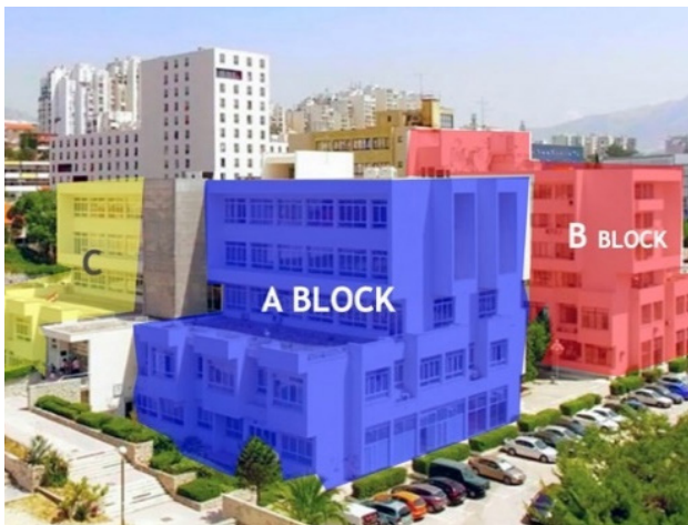
A, B and C-Blocks of Faculty of Civil Engineering, Architecture and Geodesy, University of Split.
